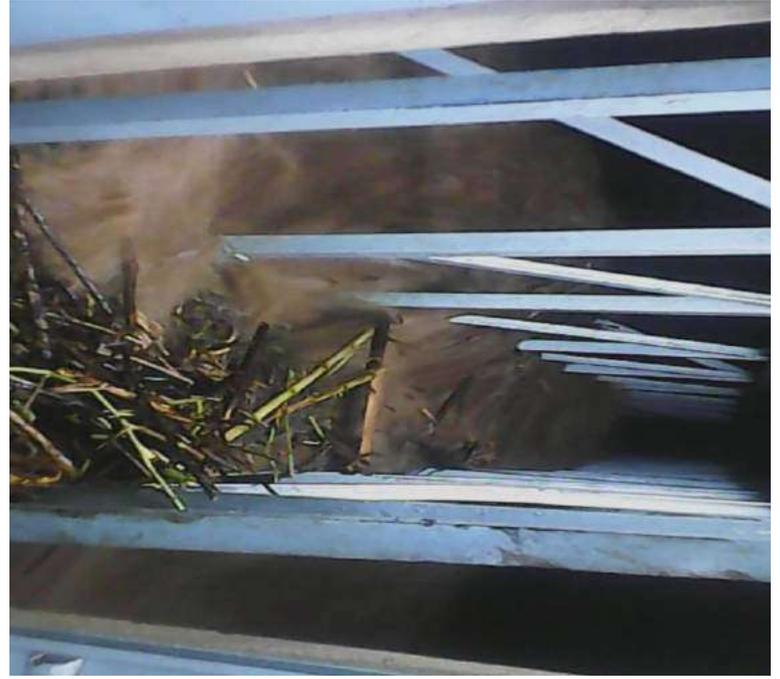
**Fig2. Clogging at Ihwa intake**
