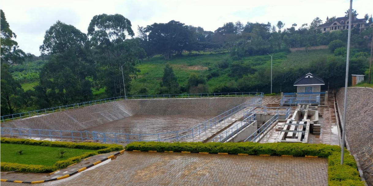
The new and operational King'ong'o Pumping Station
