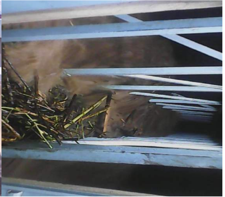
Fig2. Clogging at Ihwa intake
