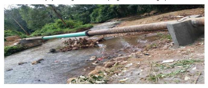
Fig1: Completed repair works at Chania River sewer crossing.
