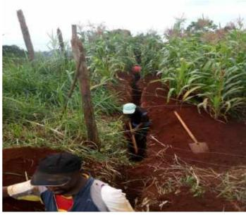
Trenches for laying pipes dug during the pipe upgrade in Kiganjo and Wambugu farm
