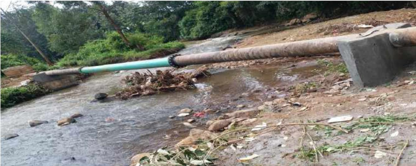
**Fig1: Completed repair works at Chania River sewer crossing.**
