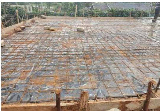
Fig3. Pipe Store foundation in Kamakwa
