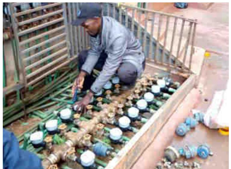
NYEWASCO NRW technical team Conducting a leak detection exercise and customer meter replacement
