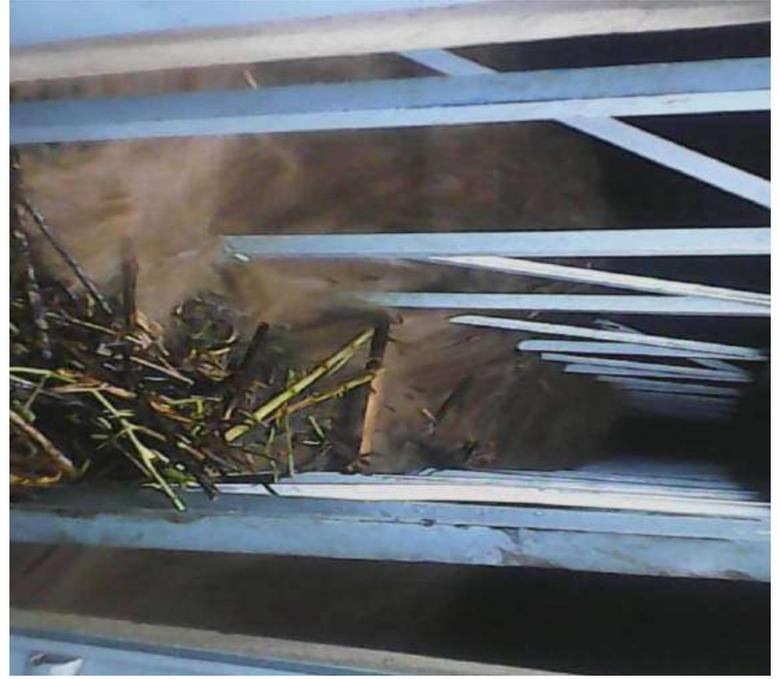
**Fig2. Clogging at Ihwa intake**
