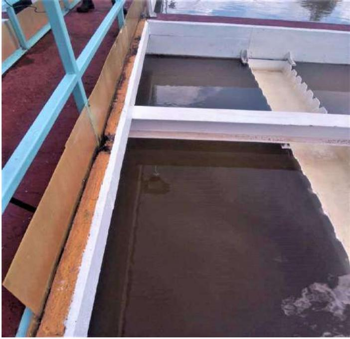
**Fig1. Highly turbid water at the treatment plant**
